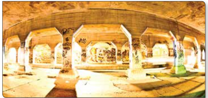
Krog Tunnel: The epicenter of debate.
