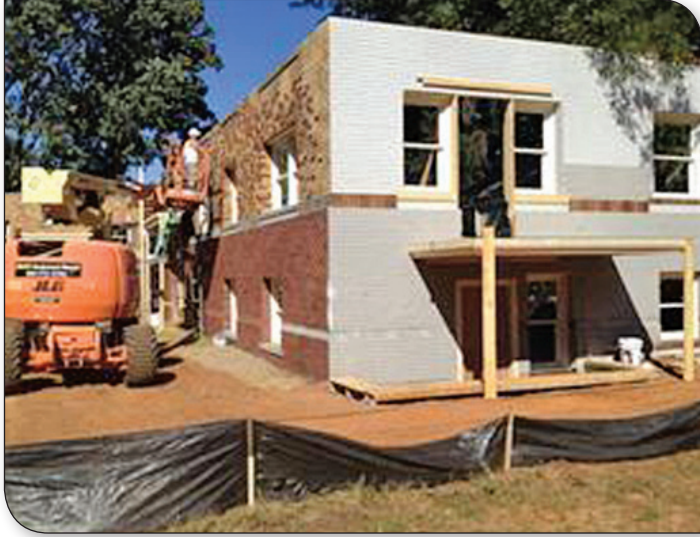
Set construction at Pearl and Kirkwood.
