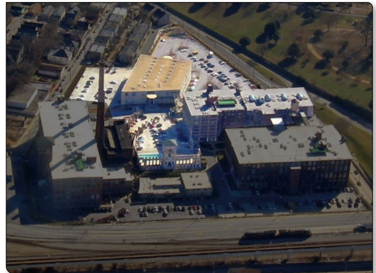
Fulton Cotton Mill Lofts (highlighted area) and The Stacks.
