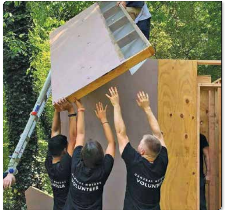
The Mad Housers volunteers building a home for a homeless person.
