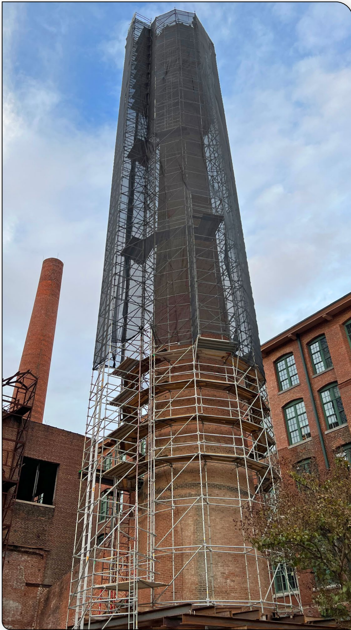
Work is underway to ensure our stacks stand for another 150 years.
