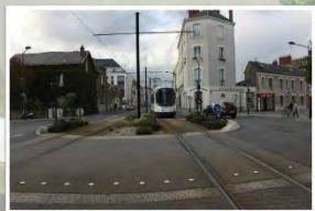
Transit Right of Way Shared Space, Nantes, France
