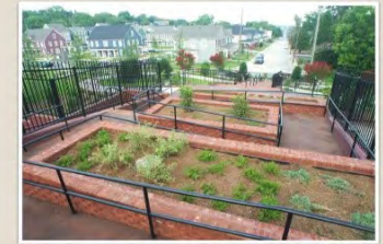
Hazel St Pedestrian Bridge, Macon, GA
