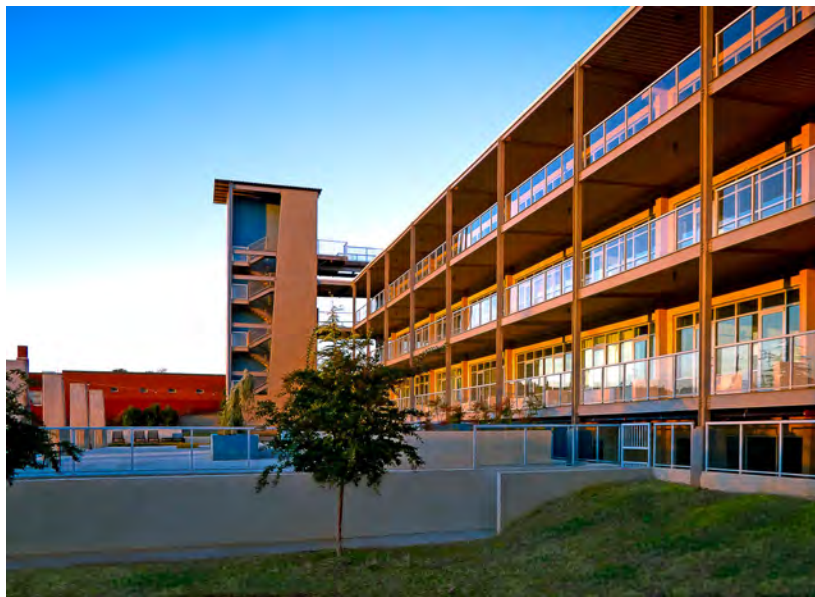
Figure 14. Lofts at Reynoldstown Crossing Phase 1
